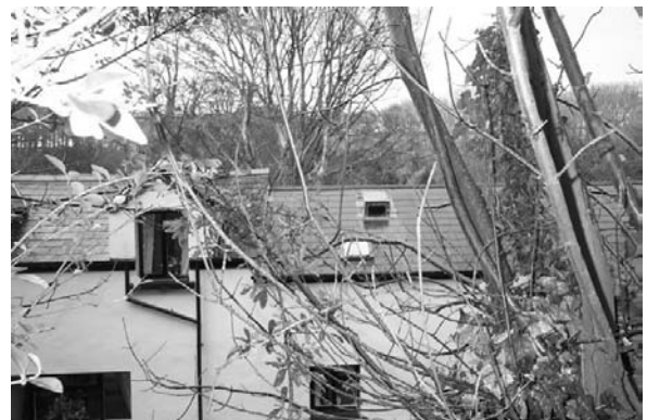
Figure 9.7.3 The roof in 2004, showing the current bats' entrance
